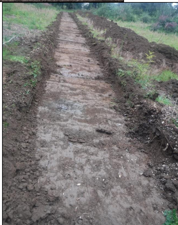
Plate 11.10 T24 from south
